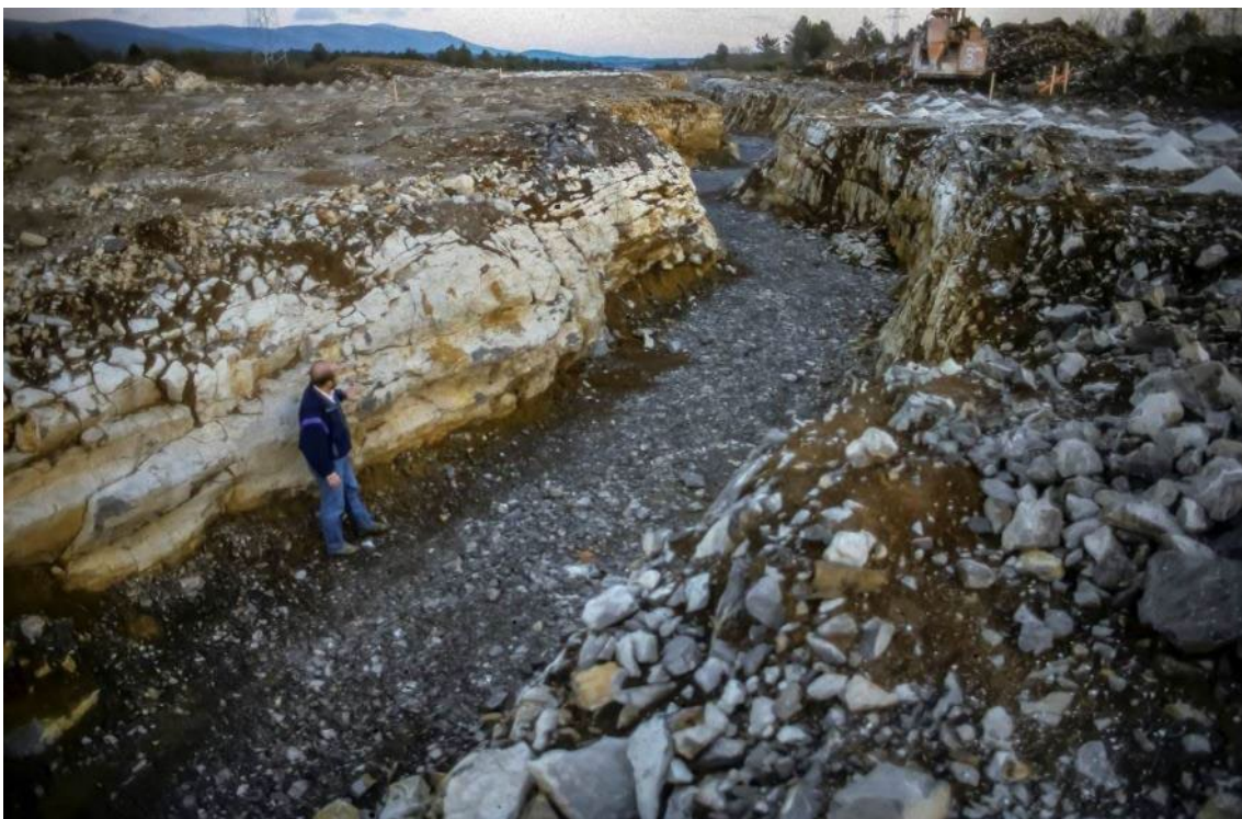
The route of the same motorway in Slovenia runs over what was originally a sediment-filled unroofed cave. Co-operation between the constructors and the Karst Institute in Postojna ensured that the cave was carefully documented before being filled with aggregate and sealed to reduce the risk of collapse. Photo by John Gunn.
