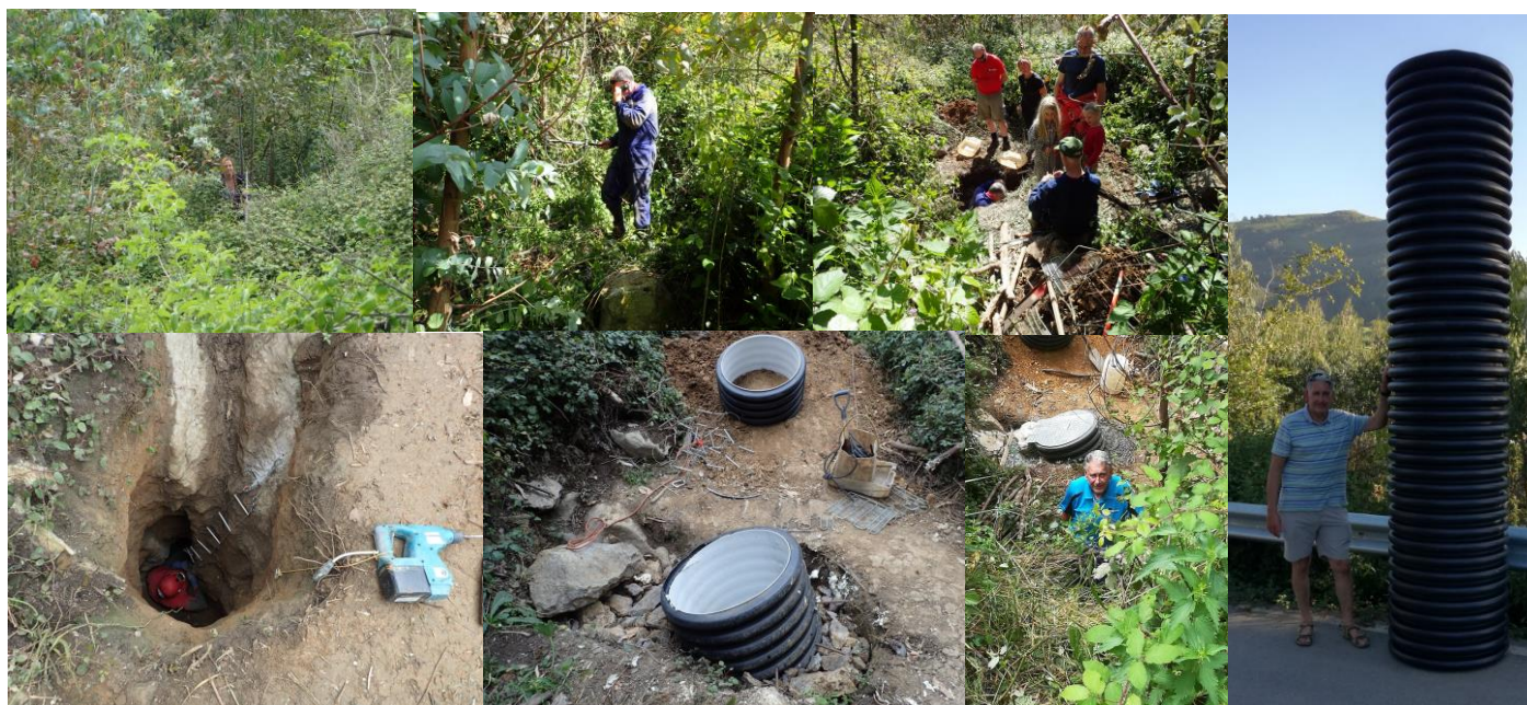
SubPhone Entrada (4536) – locating spot above SubPhone station in cave, digging, installing tube and concreting round the fitted lid
